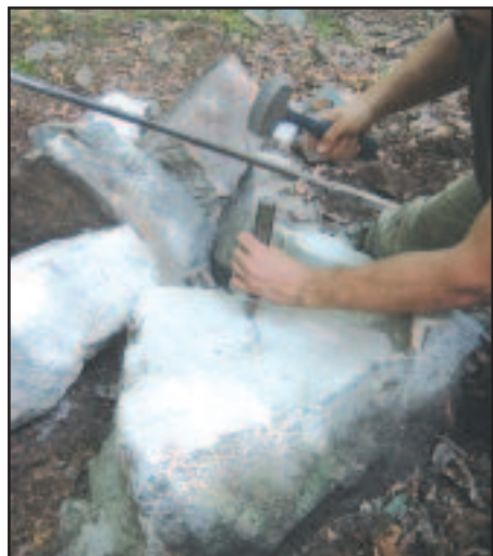
Learn to prepare rocks for use in crib walls and trail paving at Trail U.
