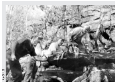
Larry Wheelock attended. Focusing on a variety of winching techniques, and analysis of the differing types of set-up for a winching system, participants—under the watchful eye of trainer Peter Jensen, a professional trails consultant from Massachusetts—applied learned skills to stockpile rocks in preparation for an upcoming trail work project on Breakneck Ridge, site of the training. In November, East Hudson Trail Crew members under crew chief Bernie Stringer began to apply their skills when they installed 20 of the stockpiled rocks into place as steps. Above, trainer Peter Jensen (left), oversees "students" John Graham, Walt Daniels, and Larry Wheelock as they guide a quarried stone along the highline.
